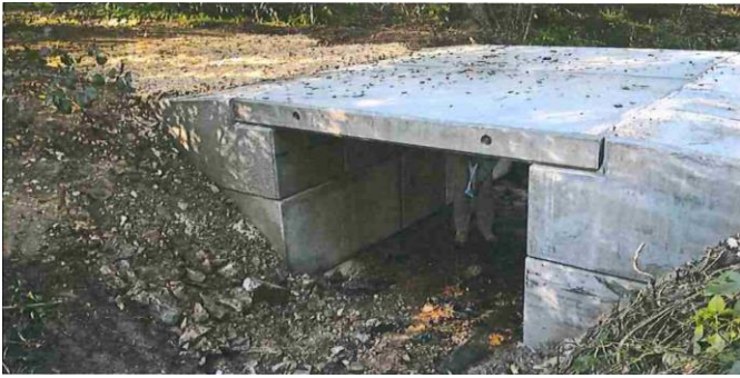
Figure 6 – Ponceau de franchissement, © ONF – Frédéric Sassard
